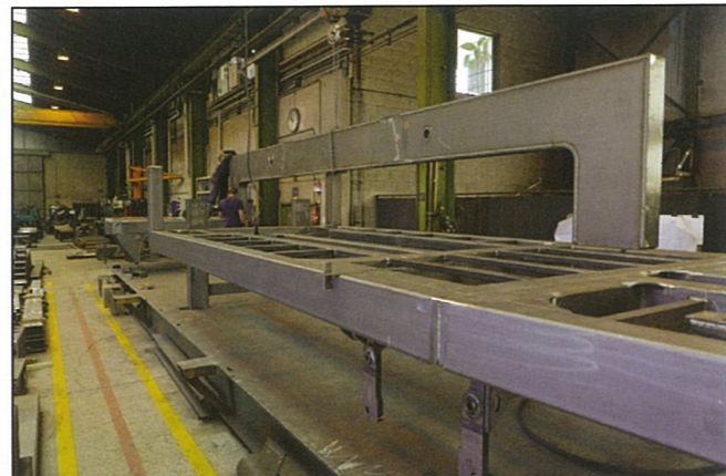
Fig. 3: As many components were to be upgraded, the main frame of the 08-16/90 tamping machine had to be re-designed and re-built, which took place at Plasser & Theurer in Linz, Austria – this highlights the importance of a close collaboration between machine service company and manufacturer
