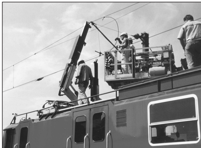
Fig. 7: Cable holding unit in operation during bracket work
