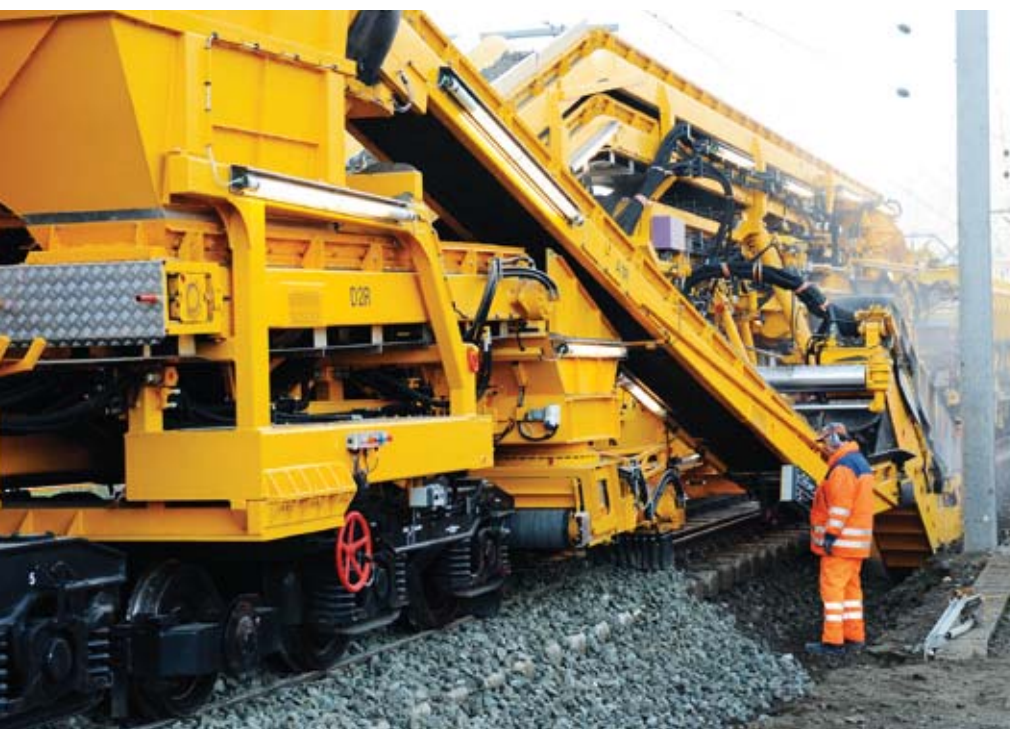
FIG. 1: Ballast cleaning in turnouts using the URM 700
