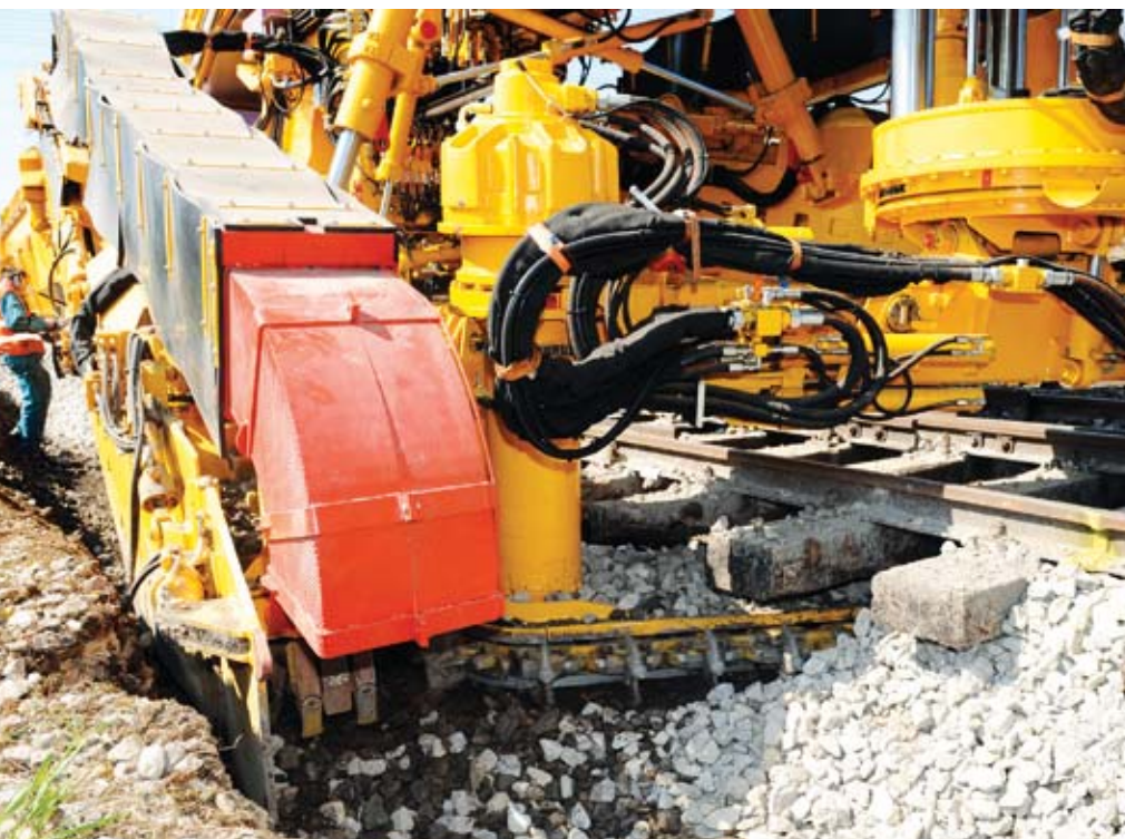
FIG 5: Excavating chain and sword of the URM 700 in operation
